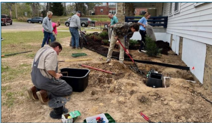
Students and volunteers spread mulch while Jacob Laughlin completes the irrigation system. Photo by Diane Peterson.
